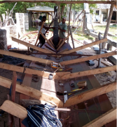
Build a temporary wooden structure to shape the hull
