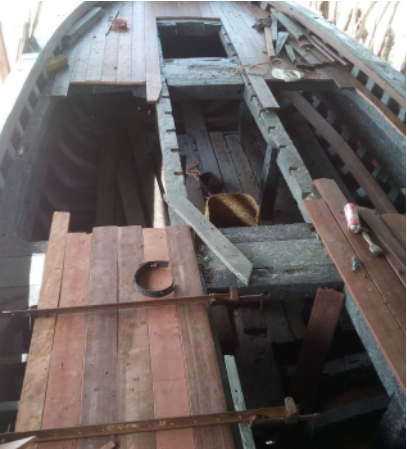
Make plank decking
